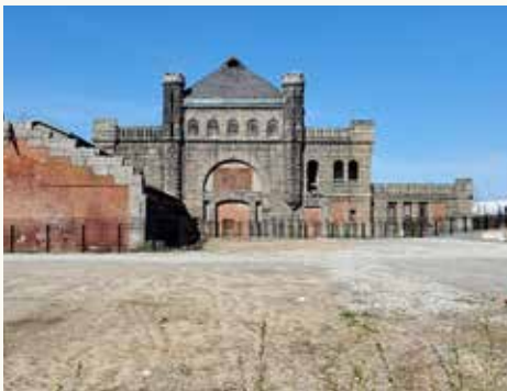
2012 Acquire Pumping Station
