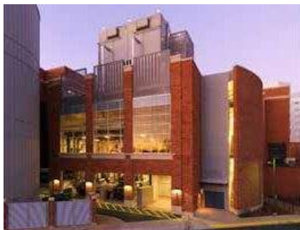
South Chiller Plant, University of Virginia. Leers Weinzapfel Associates
